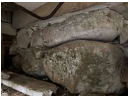
Above: Basalt foundations
