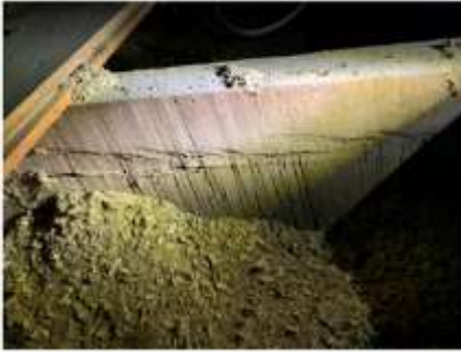
Left: Pit sawn joist and early sawdust insulation
